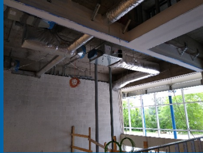
Insulate Duct and Install Steel for Lift at Entry
