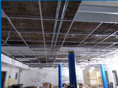
Install Ceiling Grid and Lights in Cafeteria & Kitchen
