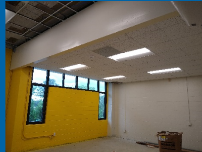
Begin Install of Ceiling Tiles at Building 2010
